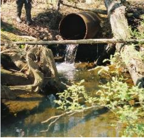
Figure 7-3. Examples of pipe outfall failure.
