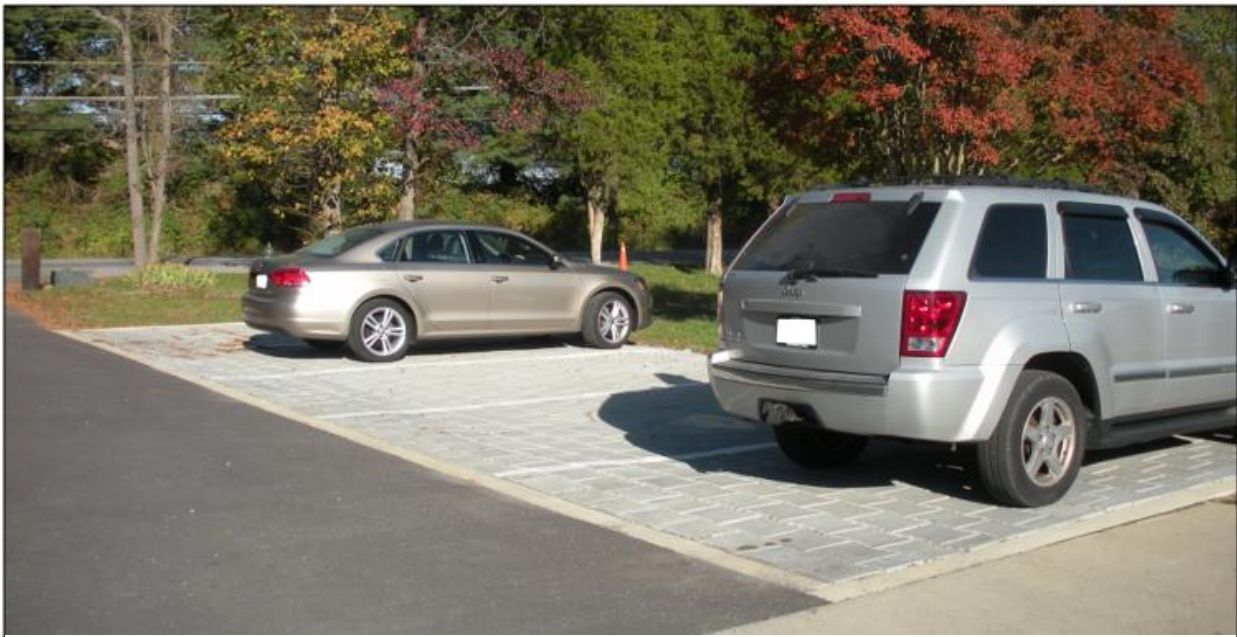
Permeable pavement is one way to treat runoff from impervious parking lots.
