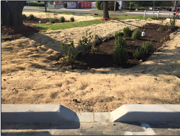
Bioretention facilities (above) and permeable pavement (right) installed by the CWP as part of the Alternative Compliance Program.
