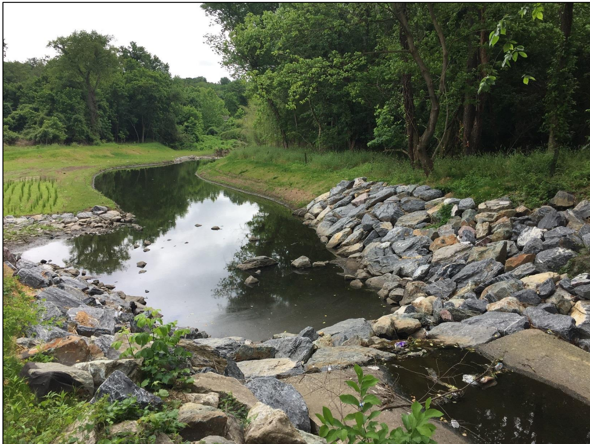
Recently completed stream restoration project. Rocks were used to stabilize the banks and fresh vegetation was planted along both banks.
