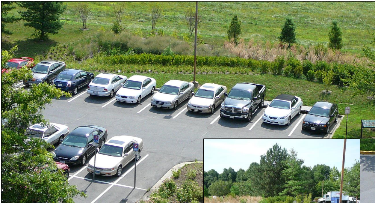
Aerial and ground-level view of bioretention facility collecting runoff from parking lot at County office building in Largo.
