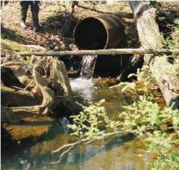
Figure 7-3. Examples of pipe outfall failure.
