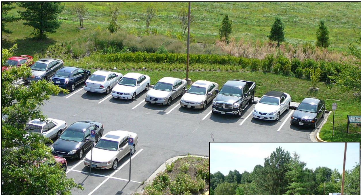
Aerial and ground-level view of bioretention facility collecting runoff from parking lot at County office building in Largo.
