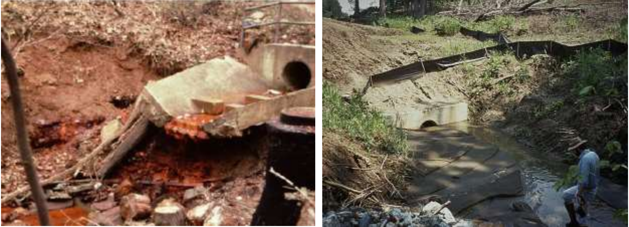
Figure 5-6. Examples of pipe outfall failure.
