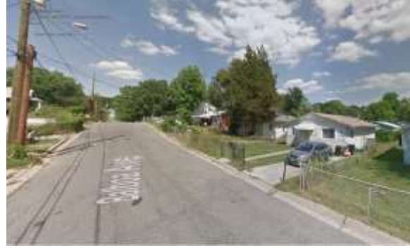
Urban closed section with curb and gutter but no sidewalk: Capitol Heights–Balboa Avenue.
