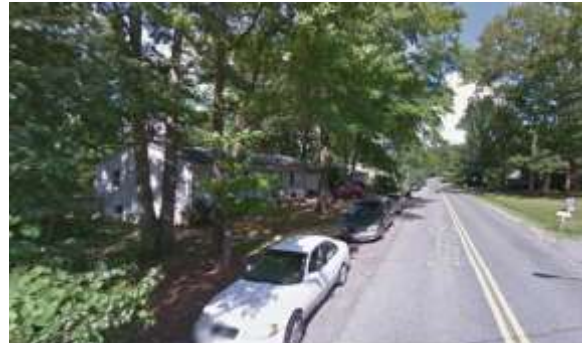
Suburban open section with no curb, gutter, or sidewalk: Glendale–Dubarry Street.
