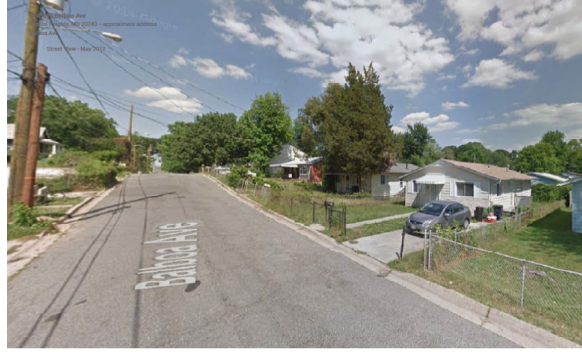
Urban closed section with curb and gutter but no sidewalk: Capitol Height–Balboa Avenue.
