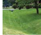
Swales and other bioretention practices filter runoff from roads and other impervious surfaces.
