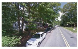
Suburban open section with no curb, gutter, or sidewalk: Glen Dale–Dubarry Street.
