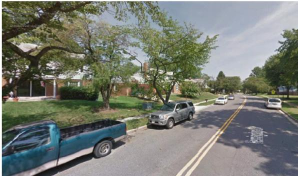
Suburban closed section with curb, gutter, and sidewalk: Kettering-Herrington Drive.
