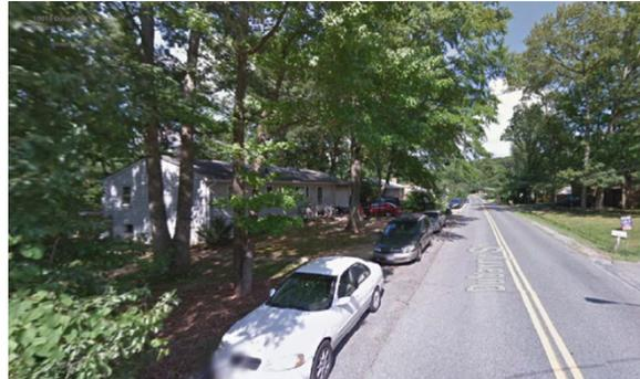
Suburban open section with no curb, gutter, or sidewalk: Glen Dale-Dubarry Street.
