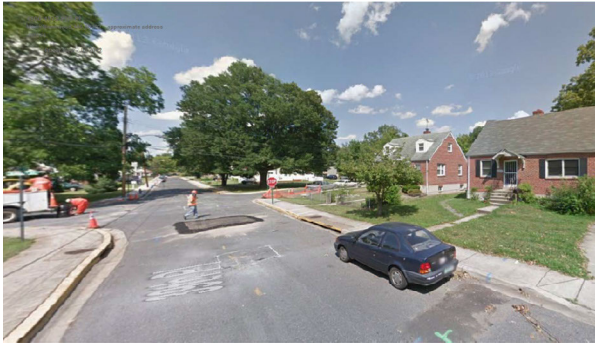
Urban closed section with curb, gutter, and sidewalk: Mt Rainier–39th Place.
