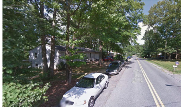
Suburban open section with no curb, gutter, or sidewalk: Glen Dale–Dubarry Street.
