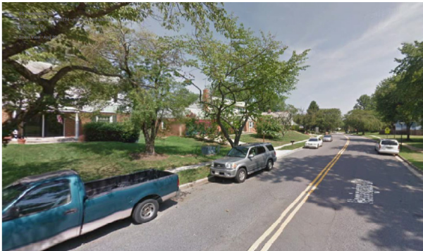
Suburban closed section with curb, gutter, and sidewalk: Kettering–Herrington Drive.
