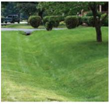
Swales and other bioretention practices filter runoff from roads and other impervious surfaces.
