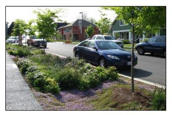
Above: Bioretention in a right-ofway makes this a green street. Below: Permeable pavement along parking lot.
