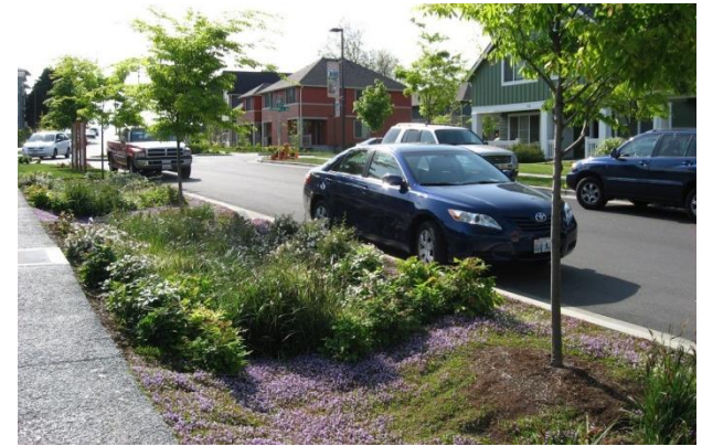
Bioretention in a right-of-way makes this a green street.
