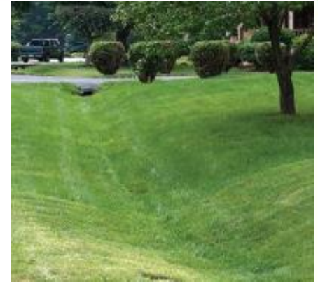
Swales and other bioretention practices filter runoff from roads and other impervious surfaces.
