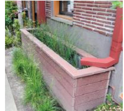
Redirecting downspouts from impervious areas to landscaped features can reduce runoff volume.
