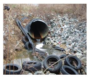
Under the restoration plans, improvements will be made to some existing stormwater infrastructure, such as this degraded outfall, in addition to the installation of new, on-the-ground management practices.
