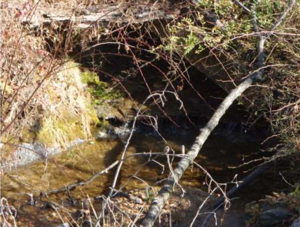
Figure C-26. Location ID 219302HC1 on February 18, 2009.
