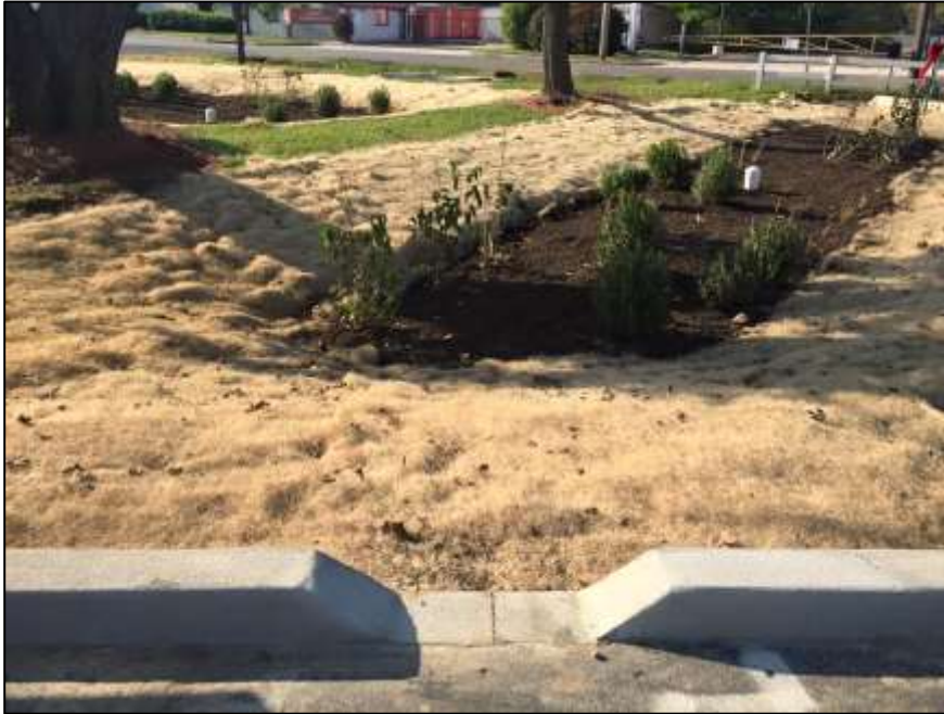
Bioretention facilities (above) and permeable pavement (right) installed by the Clean Water Partnership as part of the Alternative Compliance Program.
