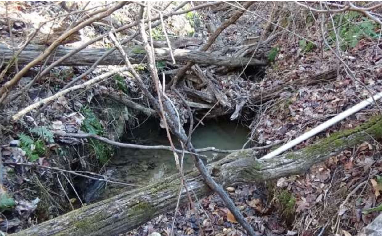
Figure C-27. Location ID 219302HC1 on February 8, 2018.
