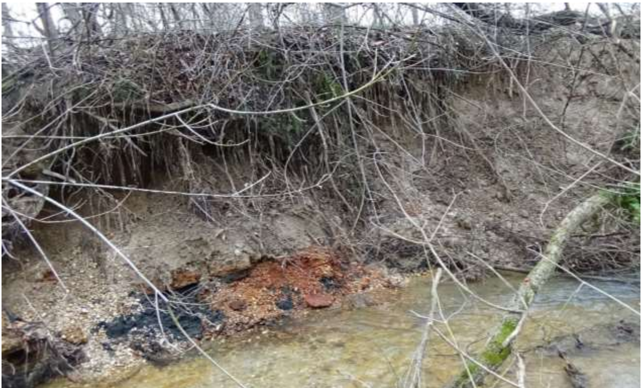
Figure C-45. Location ID 520201ES1 on March 1, 2018.
