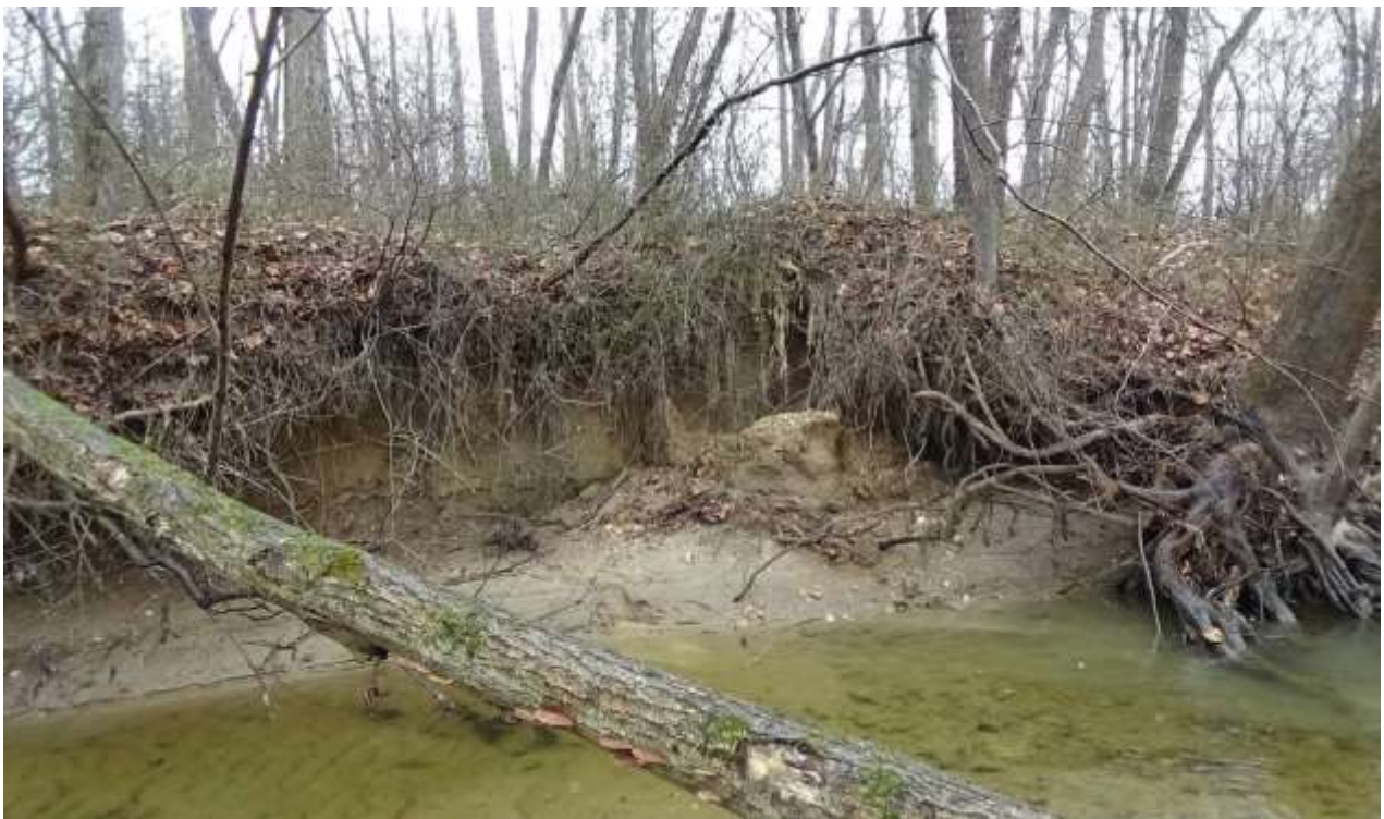
Figure C-3. Location ID 620122ES on March 1, 2018.
