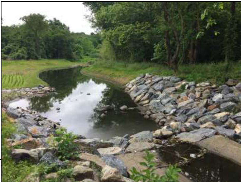
Recently completed stream restoration project. Rocks were used to stabilize the banks and fresh vegetation was planted along the left and right banks.
